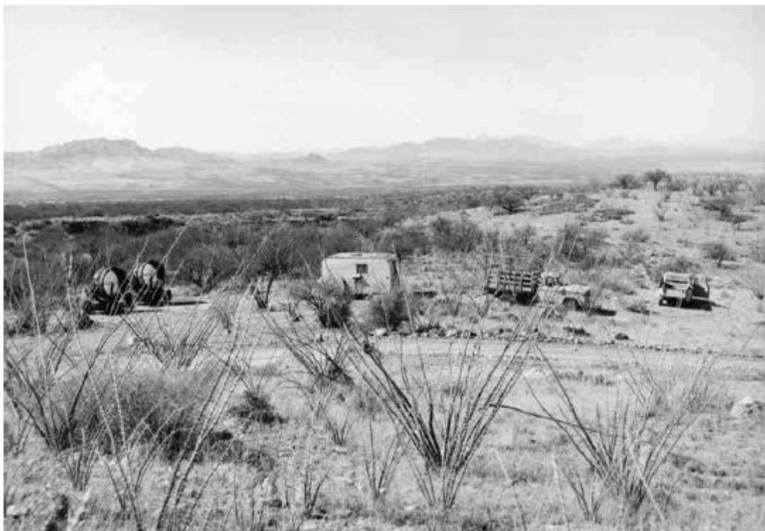
Figure 1-2. The first VHE telescope in the US, built using WWII surplus searchlights, operated in the winter of 1967-8. The site of this experiment south of Tucson, AZ is the same current location as the VERITAS observatory. [3]
