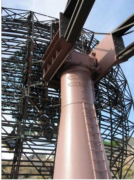
Figure 2.7: Backside of a VERITAS telescope while under construction. The frame is the OSS. Credit: The VERITAS Collaboration.
