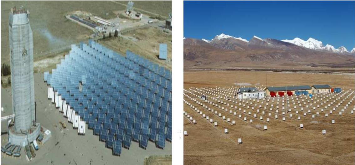
Figure 1.10: Left: The STACEE experiment consisting of solar furnace mirrors which focus Cherenkov light onto a central mirror atop the tower shown to the left. Right: The Tibet air shower array located at 4300m above sea level in Yangbajing (Tibet). The majority of the 697 scintillation detectors are shown.
