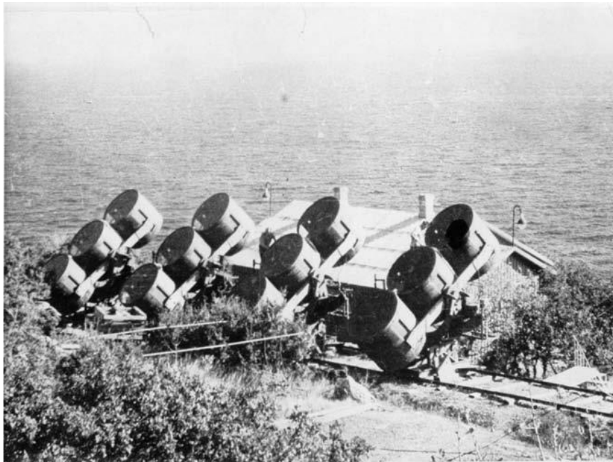
Figure 4.1: Figure 1.2 from [73]. “The Lebedev Institute experiment that operated in the Crimea, c. 1960-1964. This was the first major VHE telescope. (Photo: N.A. Porter.)”
