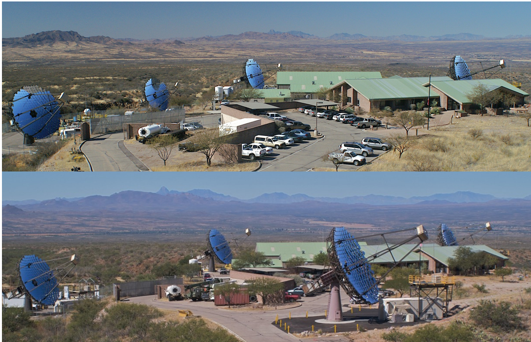
Figure 3.1.: Pictures of the VERITAS array before (top) and after summer 2009 (bottom). The relocation of one of the telescopes in summer 2009 lead to relatively uniform distances (of roughly 100 m) between the four telescopes. Image credit: VERITAS collaboration.
