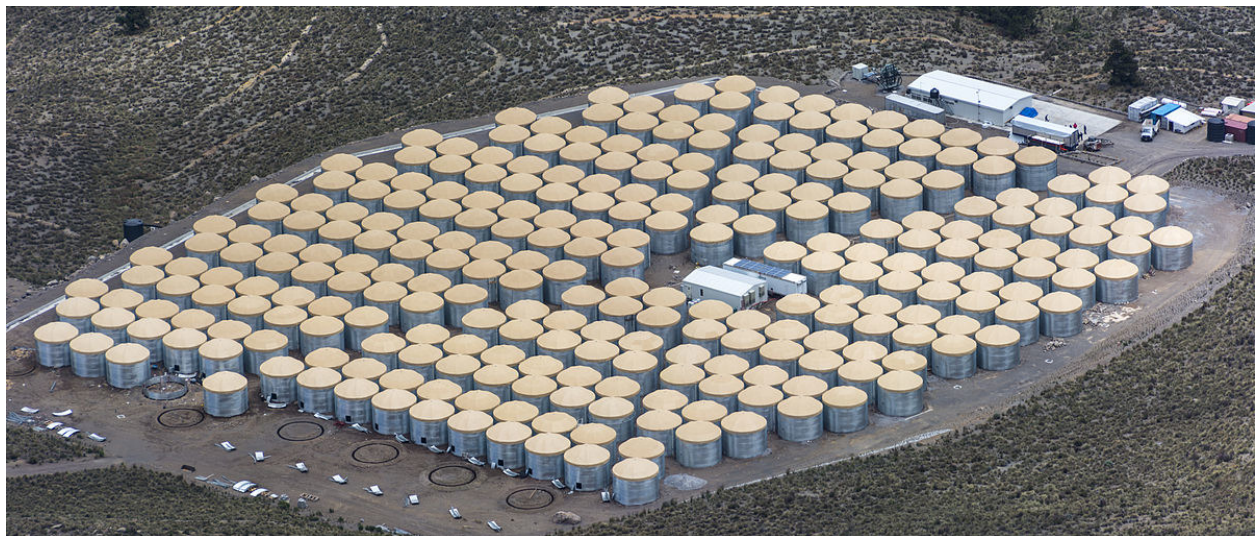
Figure 2.9: The HAWC experiment prior to completion (a few tanks in the bottom left are still missing). Image credit: “HAWC from LMT Aug 19 2014 01” by Jordan A. Goodman. Licensed under CC BY-SA 4.0 via Wikimedia Commons
